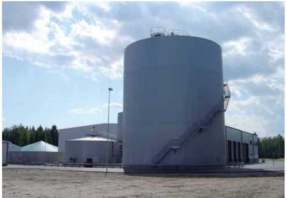
An exterior view of one of Ros Roca's AD plants, some 30 of which are now in operation across Europe.
