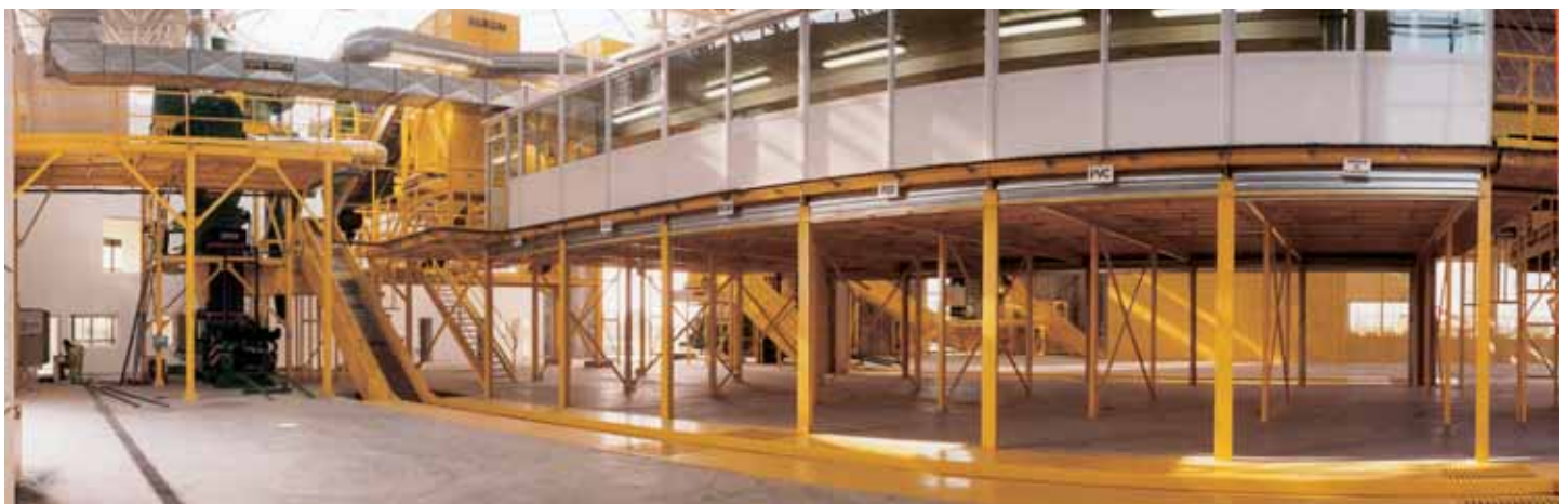
An internal view of one of Ros Roca's AD plants.
